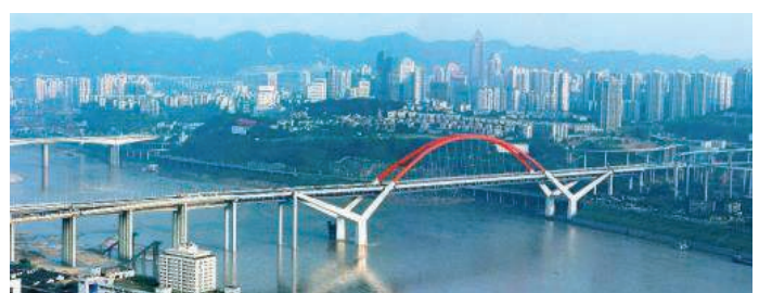
27. Łukowy most Caiyuanba Bridge [1]
