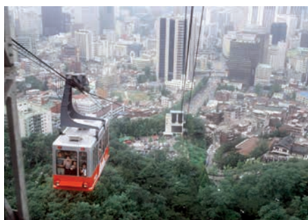
15. Kolejka Namsan Cable Car w Korei [16]
