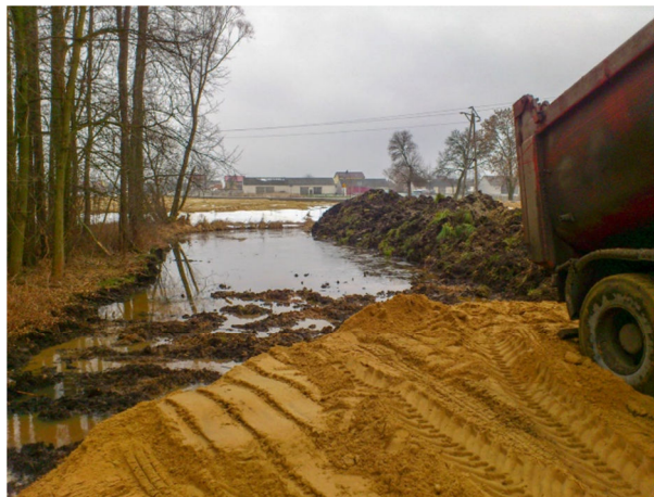
7. Replacement of low bearing soils [16]
