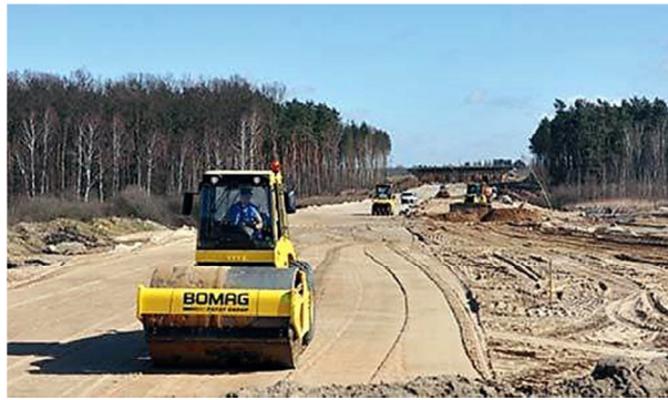
4. Mechanical compaction of the subsoil
