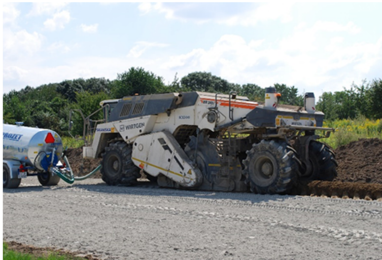
5. The process of mixing native soil with a chemical agent
