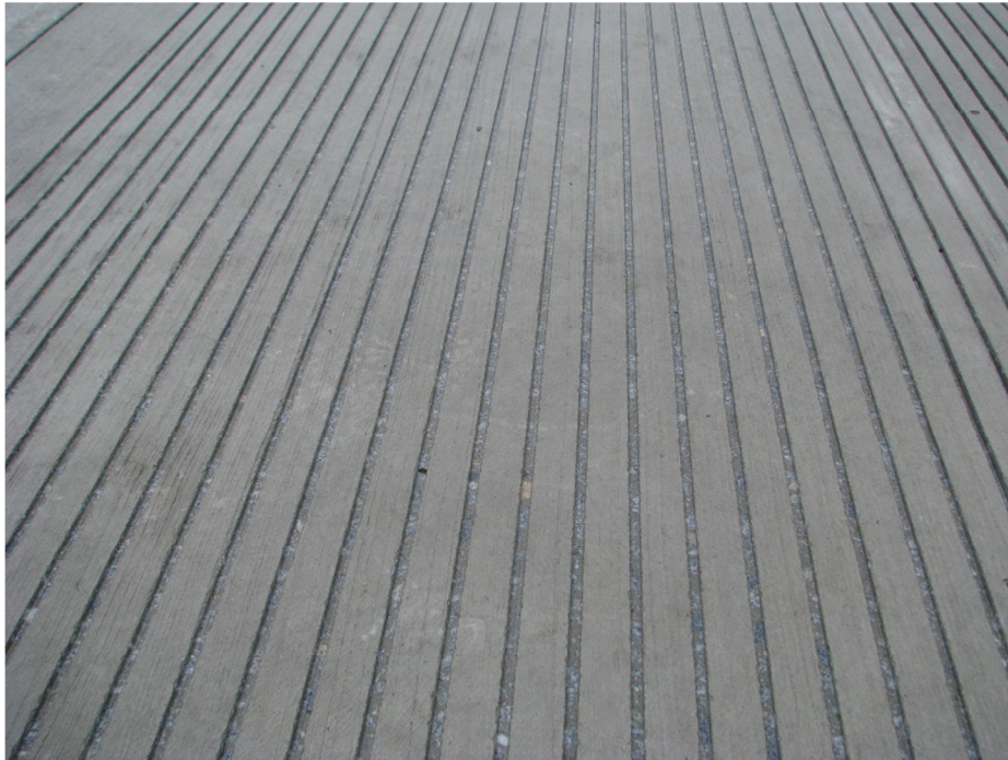
9. Texture of the pavement as a result of grooving
