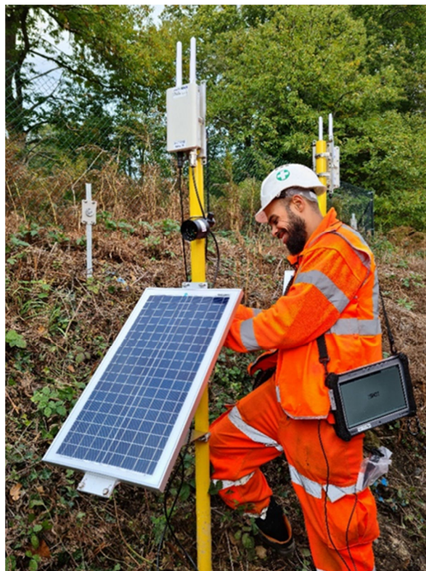
5. EdgeHub Communications Center, 4G camera and solar panel
