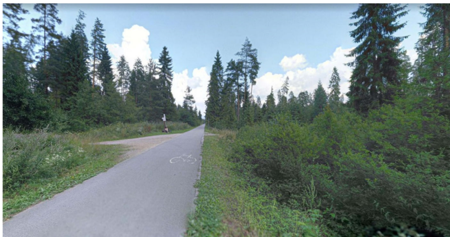
31. Former line 118 in the area of the planned Nowy Targ Bór branch post
