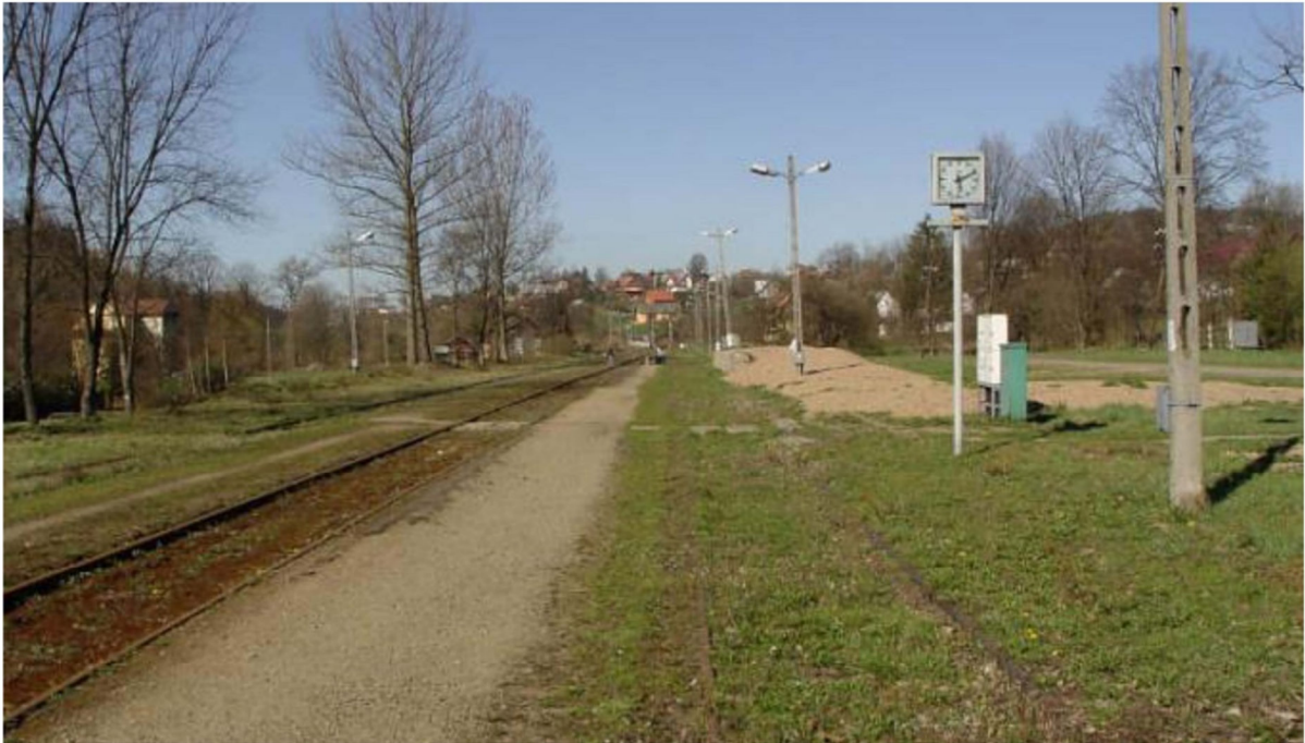
21. Rabka Zaryte station - view towards Chabowka. The beginning of the planned investment
