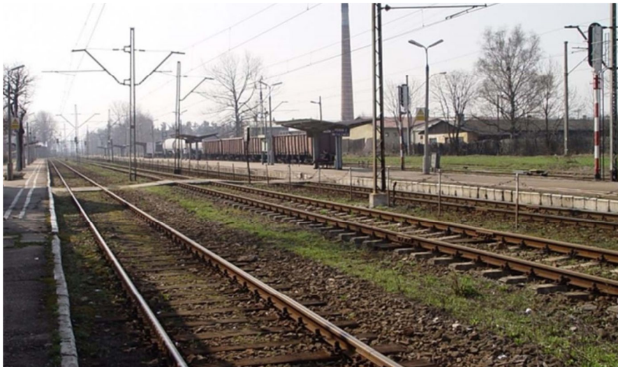
29. Nowy Targ station, view towards Zakopane
