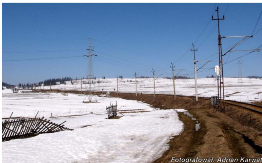
25. The Laski-Pyzówka trail. View from the Lasek side towards the planned exit of the tunnel in the W1 variant. On the left, the place where the line in variant W1 joins line No. 99
