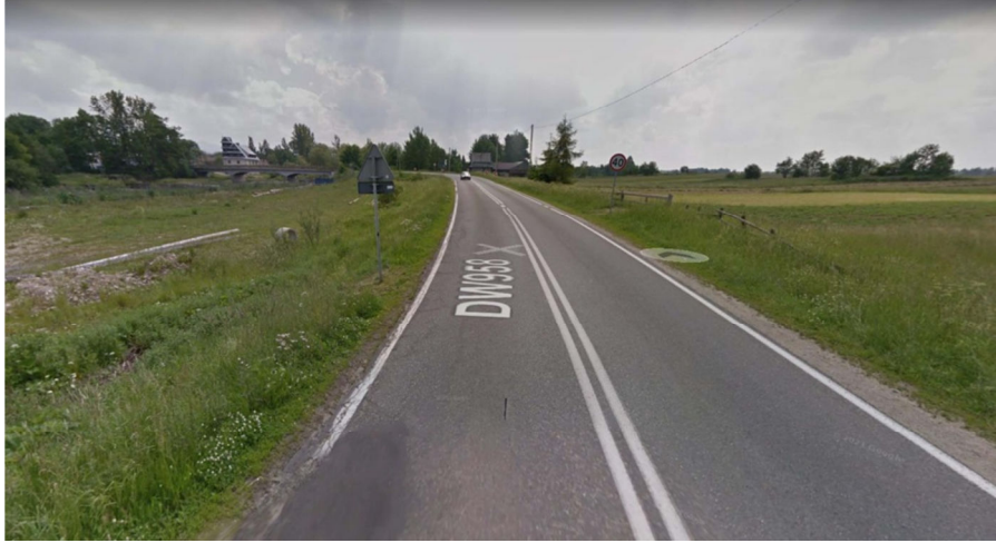
36. Infrared area of the planned bridge over the Czarny Dunajec River and the DW958 road
