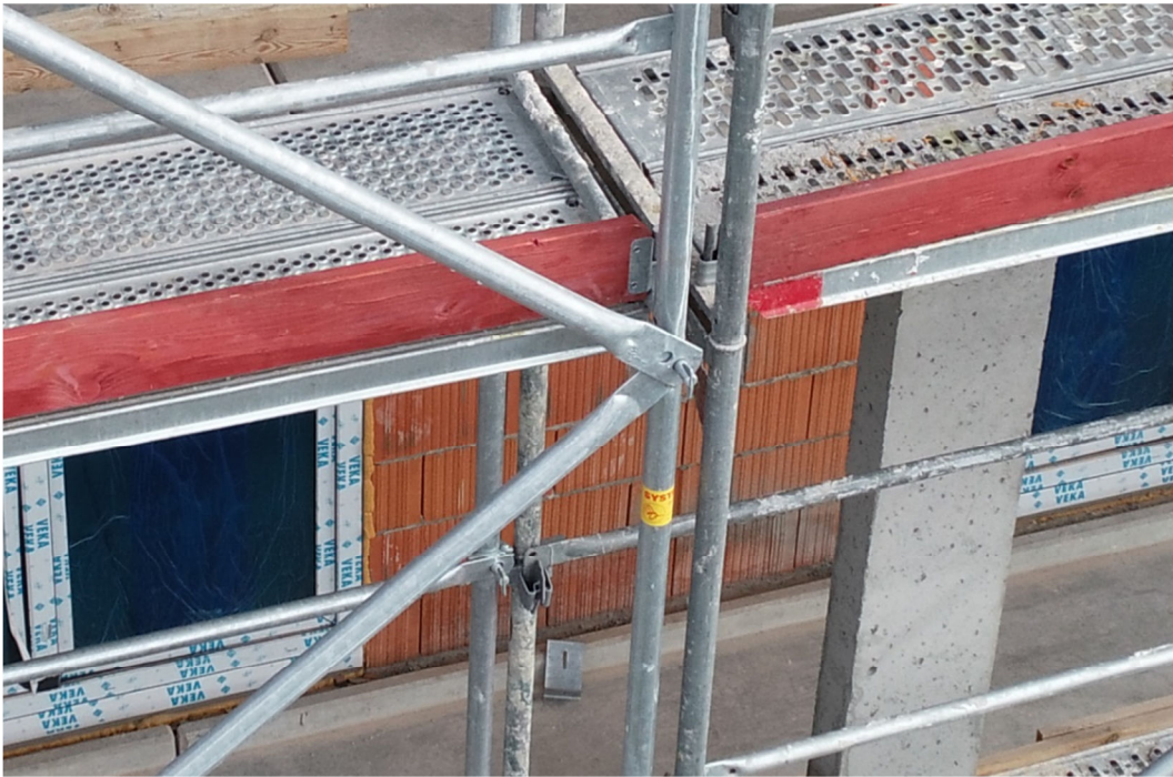
1. View of the scaffolding construction detail - connection
