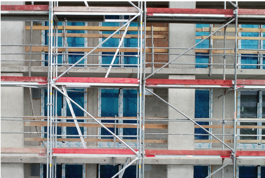
2. View of the scaffold bracing perpendicular
