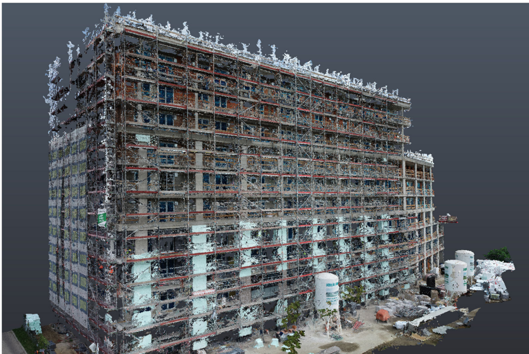
6. General view of the developed point cloud
