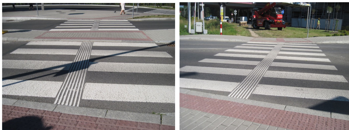
15a and 15b Modified leading lanes (older lanes) with length to curbs, Rondo Księstwa Cieszyńskiego, Cieszyn (Poland) (Photo by K. Kaperczak)
