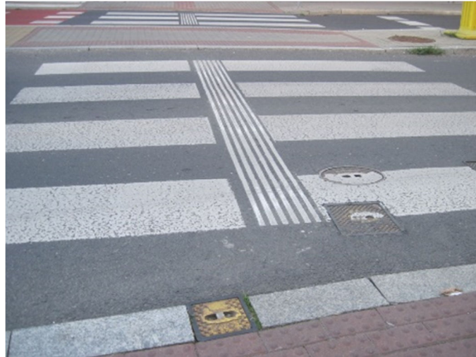
16. Modified leading lanes (newer lanes) with reduced length (only for longitudinal lanes), Rondo Księstwa Cieszyńskiego, Cieszyn/Poland (Photo by K. Kaperczak)
