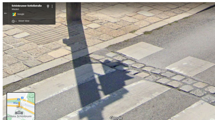
2. A leading lane made of split stone cubes - close-up, Vienna/Austria (Photo: Google)
