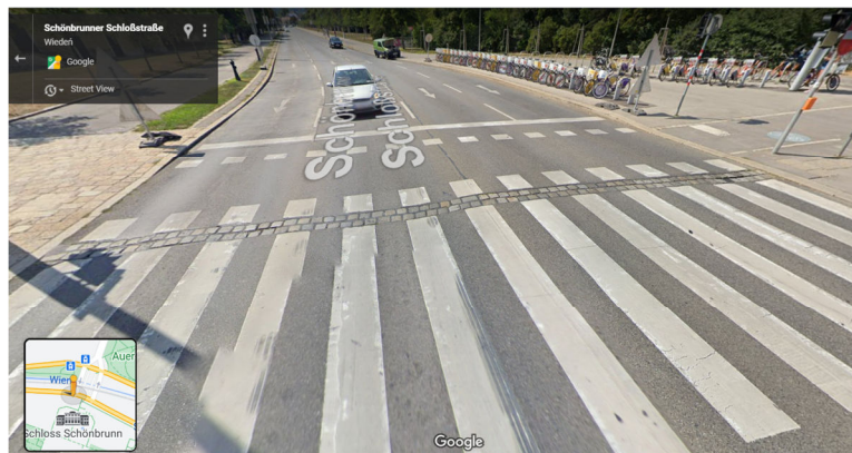
1. Leading lane made of split stone cubes - general view, Vienna/Austria (Photo: Google)
