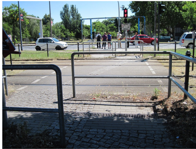
8. Stone paving lane - general view, Dresden/Germany (Photo K. Kaperczak)
