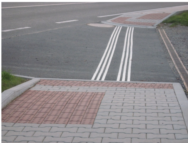
12. Independent leading lane made of chemically hardened masses, Piosek/Czech Republic - Zaolzie (Photo K. Kaperczak)
