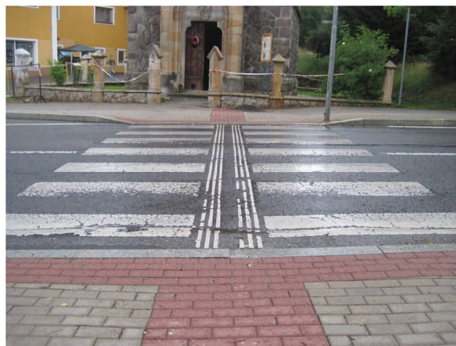
11. A leading lane made of chemically hardened masses in the "zebra" structure, Harrahov/Czech Republic (Photo K. Kaperczak)
