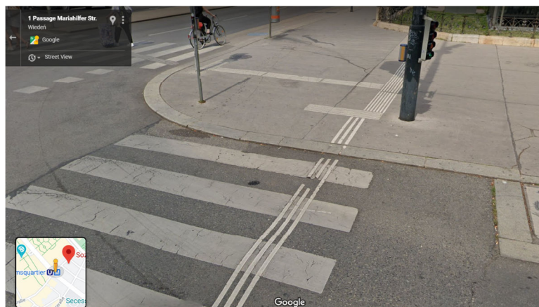
6. Leading lane made of chemically hardened masses - close-up, Vienna/Austria (Photo: Google)
