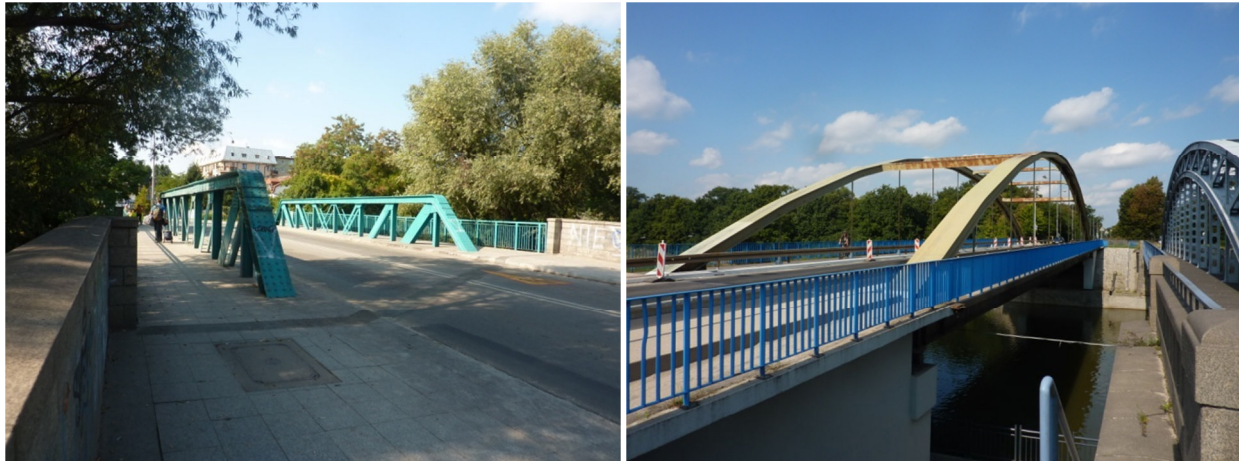
12. Examples of double-girder bridges
