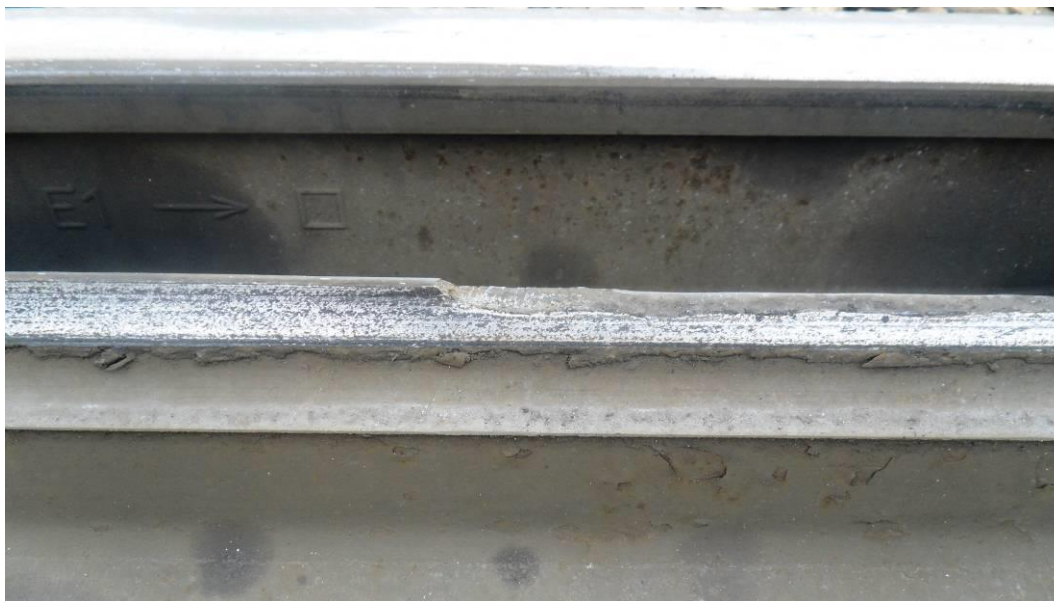
1. The chipping of the worn needle
