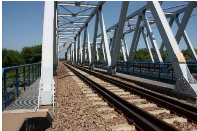
4. Truss bridge with a track laid on a ballast
