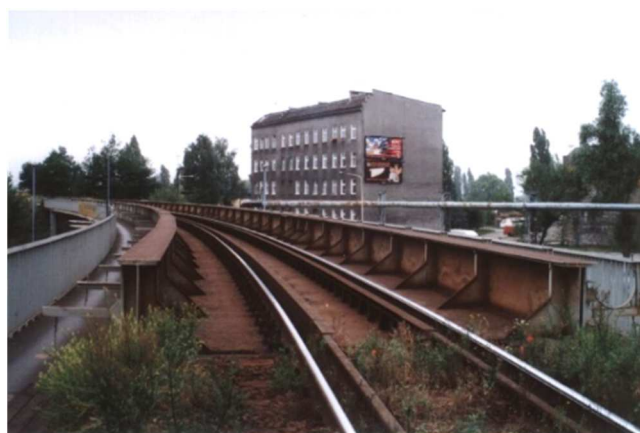
1. Overhead gantry with steel platform without ballast
