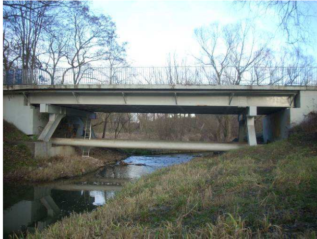
3. General view of the bridge after strengthening
