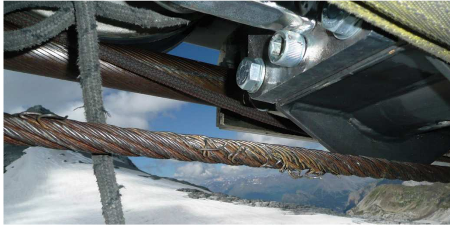
10. Cracks in wires due to fatigue corrosion [7]
