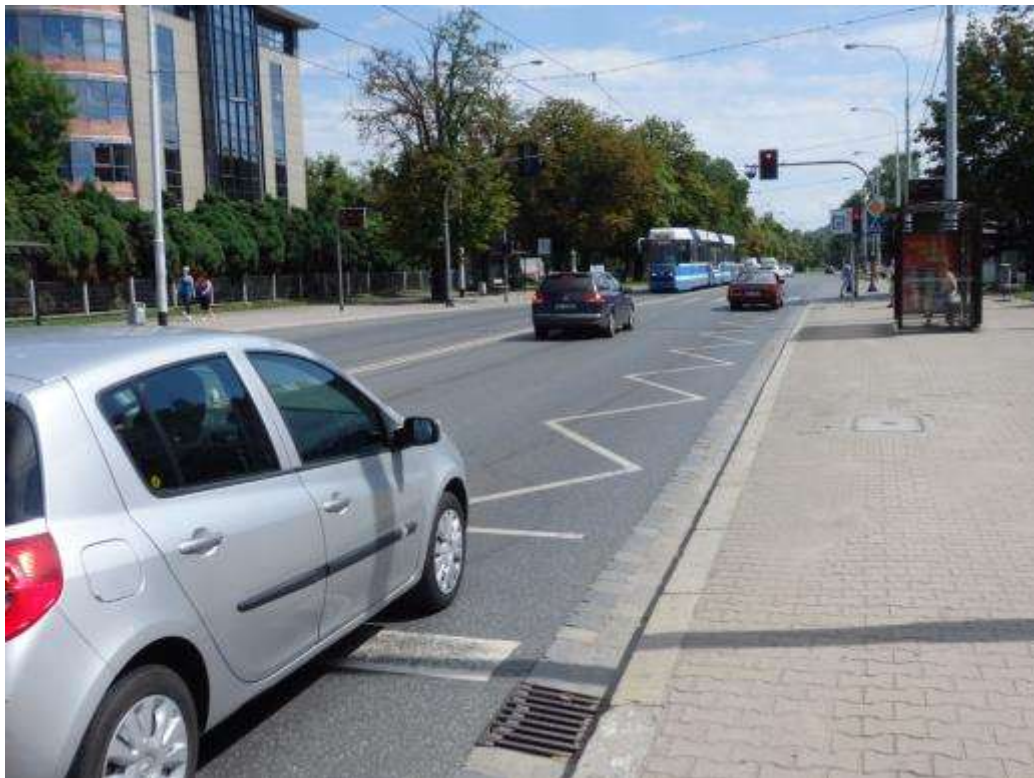
1. Tram stop without separate islands „Hutmen” at Grabiszyńska Street in Wrocław (phot. Cz. Wolek)
