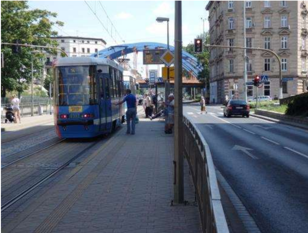
2. Tram stop with separate islands „Pereca” at Grabiszyńska Street in Wrocław (phot. Cz. Wolek)
