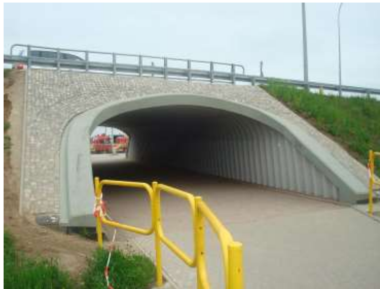
1. A view of road soil-steel structures
