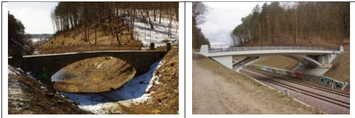
3. Demolished viaduct name of David Weiser (left) and newly built footbridge in the area of street Gomółki in Gdansk Wrzeszcz (photo by Pawel Dabrowski)
