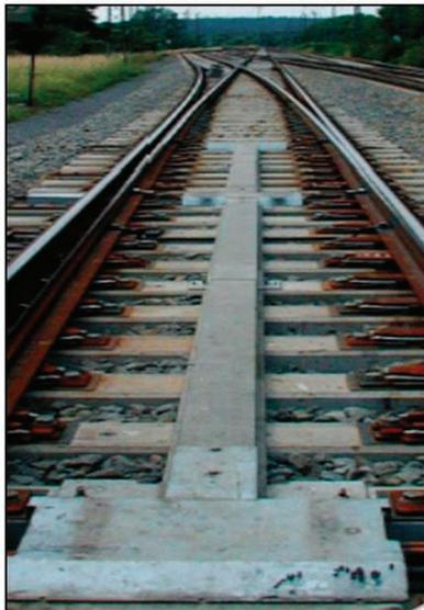
Hydraulic driven setting and locking device, concrete bearers and Vossloh fastening system
